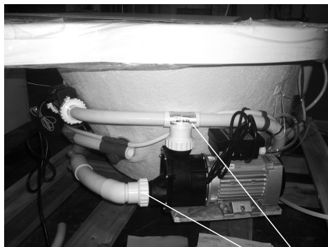
Check Connections for Leakage 检查接头处连接是否渗漏
