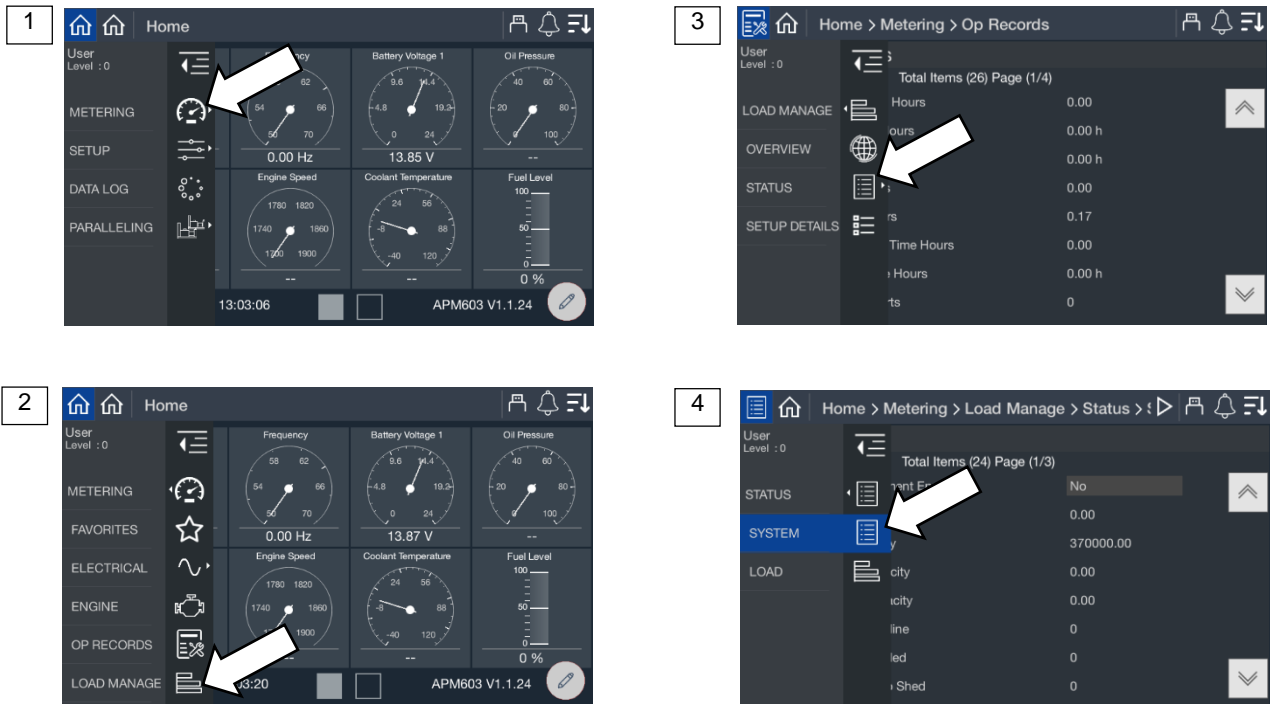
Figure 38 Metering, Load Management, Status, System
